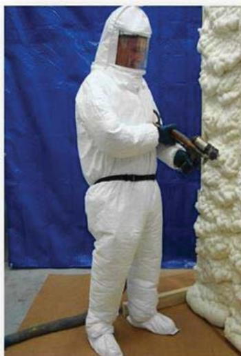
Although Personal Protective Equipment (PPE) requirements will vary depending on the type of SPF product and nature of the application, here is an example of an SPF applicator wearing proper PPE for this interior two-component high-pressure SPF installation.
